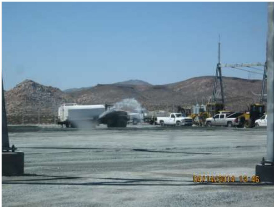
Photo 6: In accordance with MM-BIO4-A and MM-AQ-1, water trucks are utilized to minimize dust along access roads and commonly used routes within the substation boundaries.
